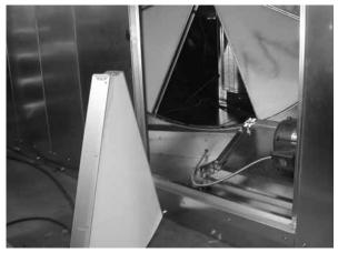
**FIGURE 29:** Wheel segment removed to allow for cleaning.
